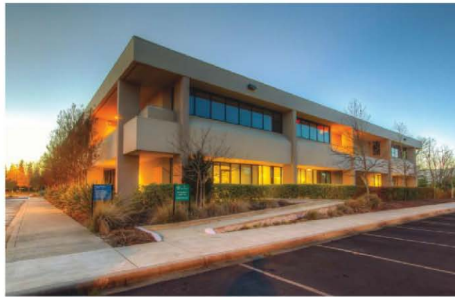
Petaluma Health Center occupies the medical office building in Rohnert Park, Calif., located at 5900 State Farm Drive.
