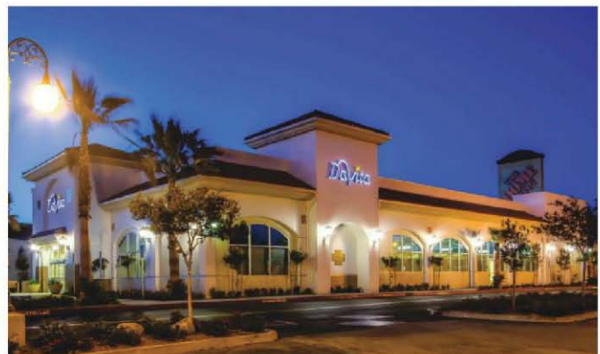
Meridian built this freestanding single-tenant building for DaVita on an outparcel in front of Home Depot in Pomona, Calif. The addition of medical services into this struggling center helped to increase traffic and breathe life into an otherwise dying center.
